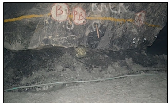
Fig. 14. Pillar failure as prompted by foot wall faults.
