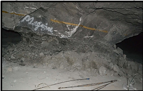
Fig. 17. Hour glassing progressive pillar slabbing.
