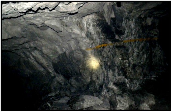
Fig. 15. Pillar failure influenced by dykes.
