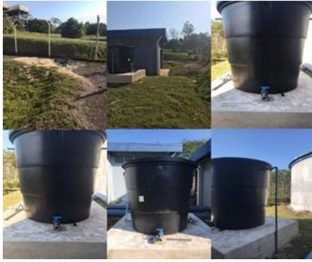
Fig. 3. Constructed water tank for dual System
