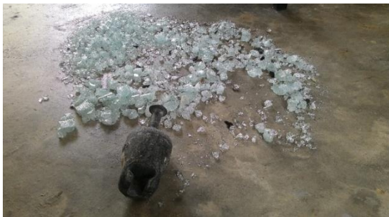
Fig. 1. Example of broken glass insulator.
